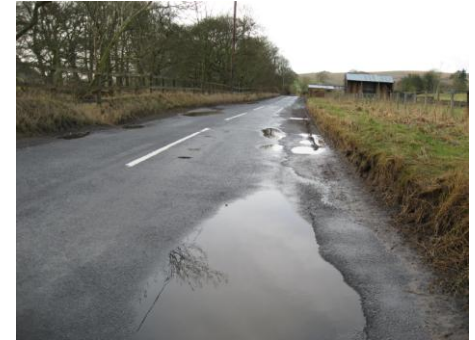
Road to Bellingham just west of West Woodburn- prone to flooding from the adjacent River Rede and frequently patched up
