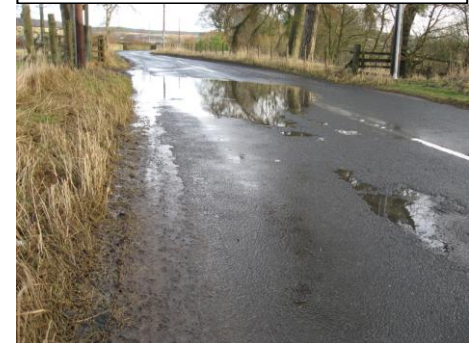
Road to Bellingham just west of West Woodburn- prone to flooding from the adjacent River Rede and frequently patched up
